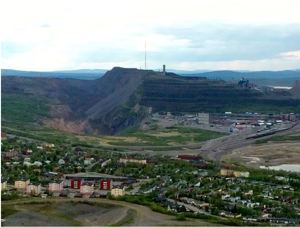
Figure 2.1: The effects of sublevel caving in Kiruna.
