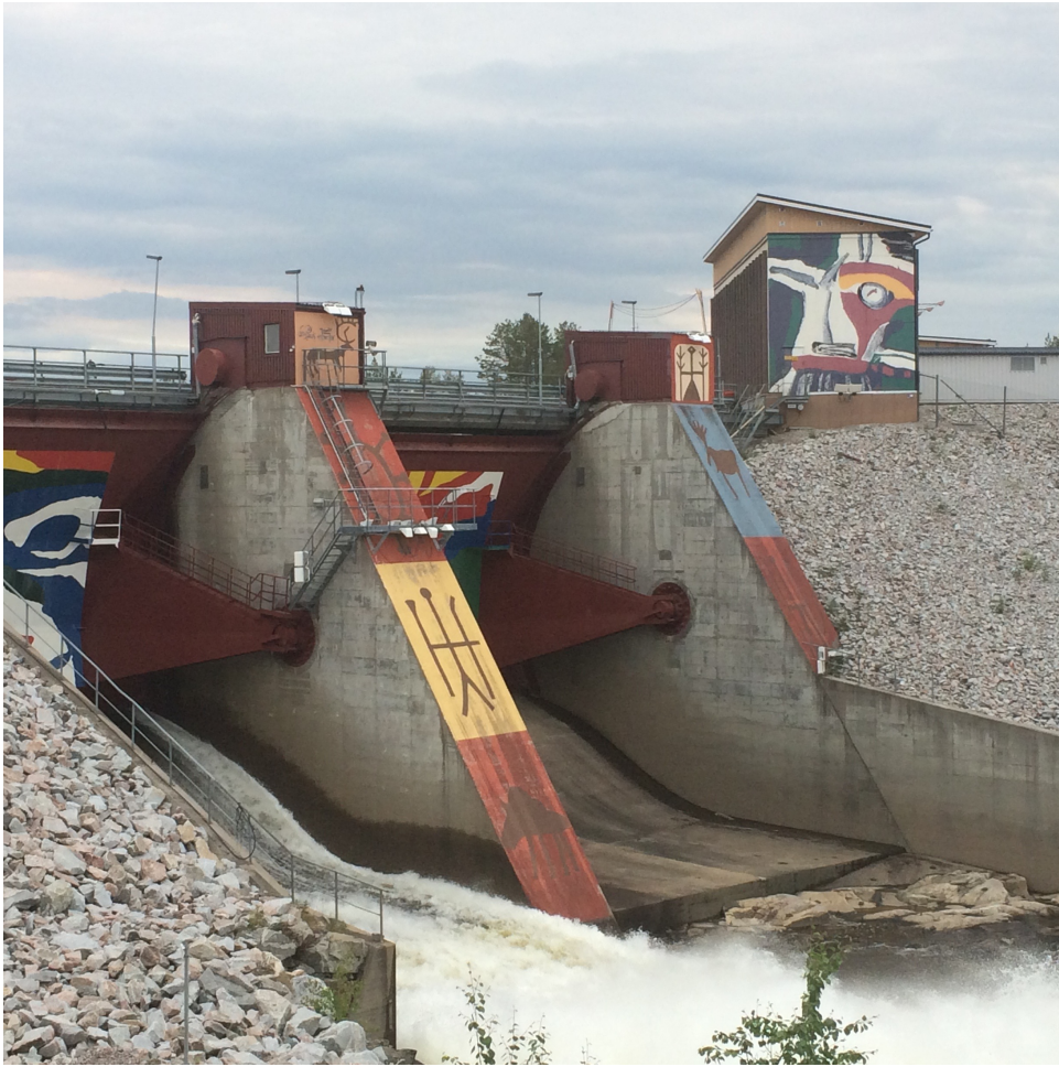
Figure 2.5: A small hydropower plant along the lilla luleälven near Jokkmokk, decorated with Sami art.
