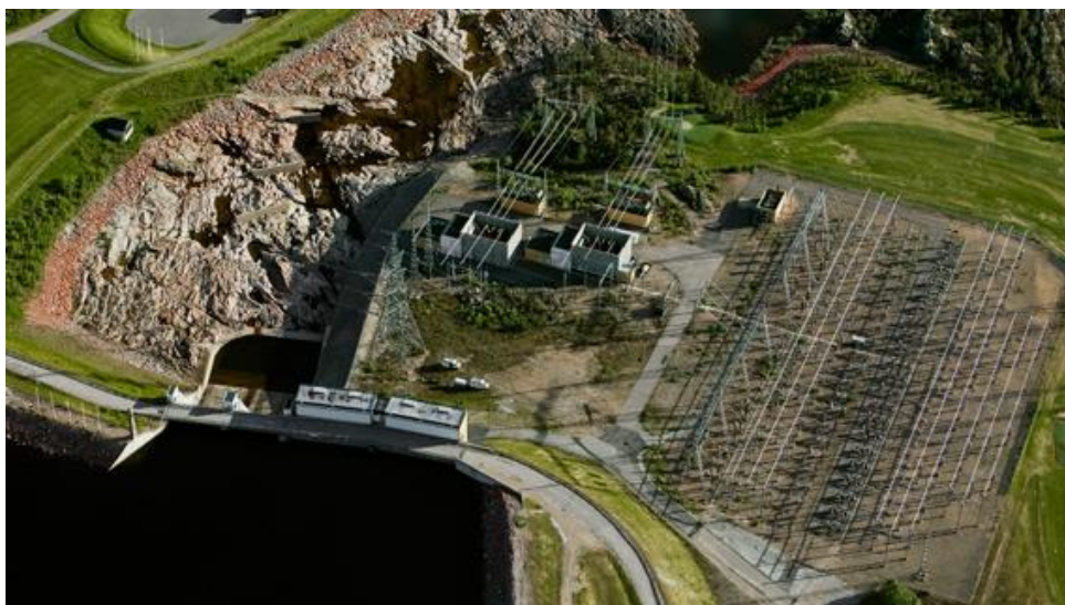
Figure 3.4: The hydropower plant at Porjus, from above. [39]
