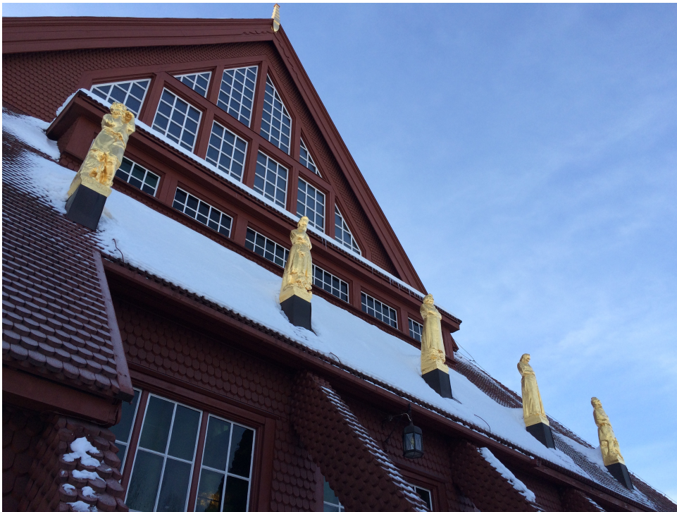
Figure 2.2: The Kiruna Church, which will be dismantled and reconstructed in New Kiruna.
